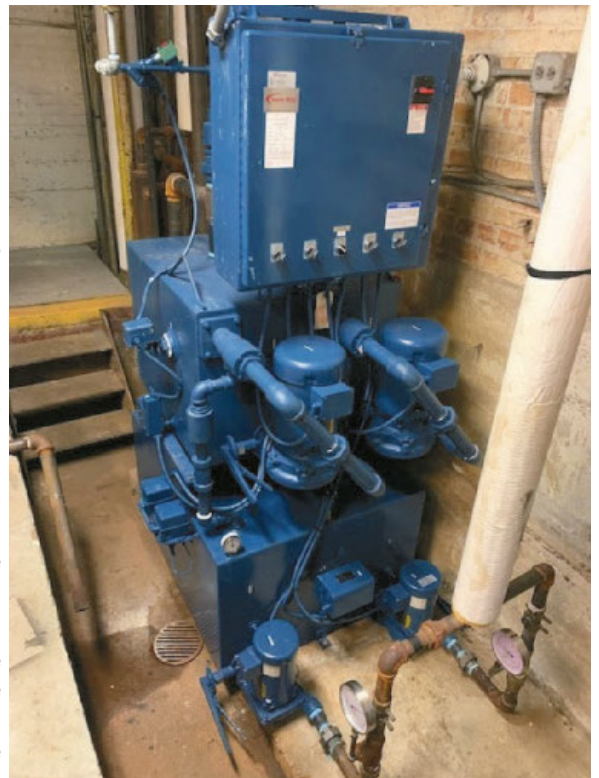
Vacuum and Condensate pump for boilers that pulls steam back from Church, Rectory, Frawley and Corrigan Buildings. The pump helps the boilers maintain even amount of steam throughout the campus heating system.
